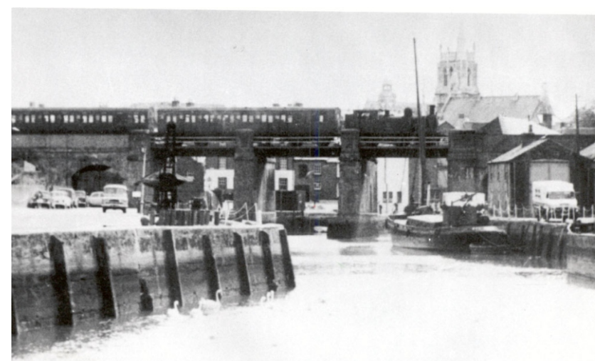
Fig. 8 Train via duct over River Medina - Isle of Wight Council Archive
