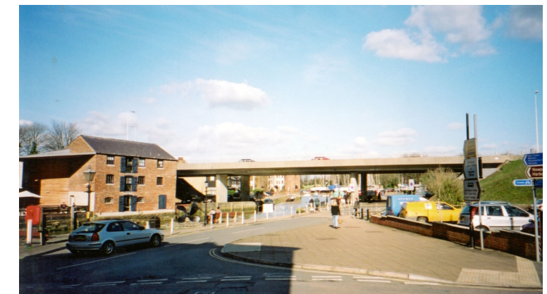
Fig. 23 The Newport Road Bridge
