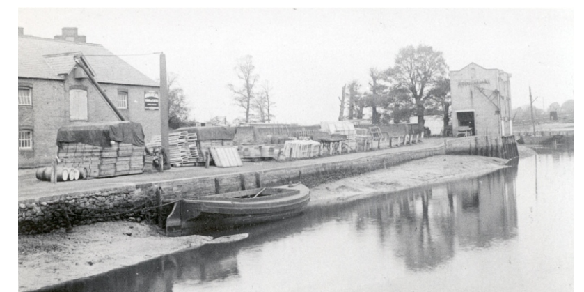
Fig. 9 View of the West quay. It is interesting to see the open space available for unloading cargo. Isle of Wight Council Archive
