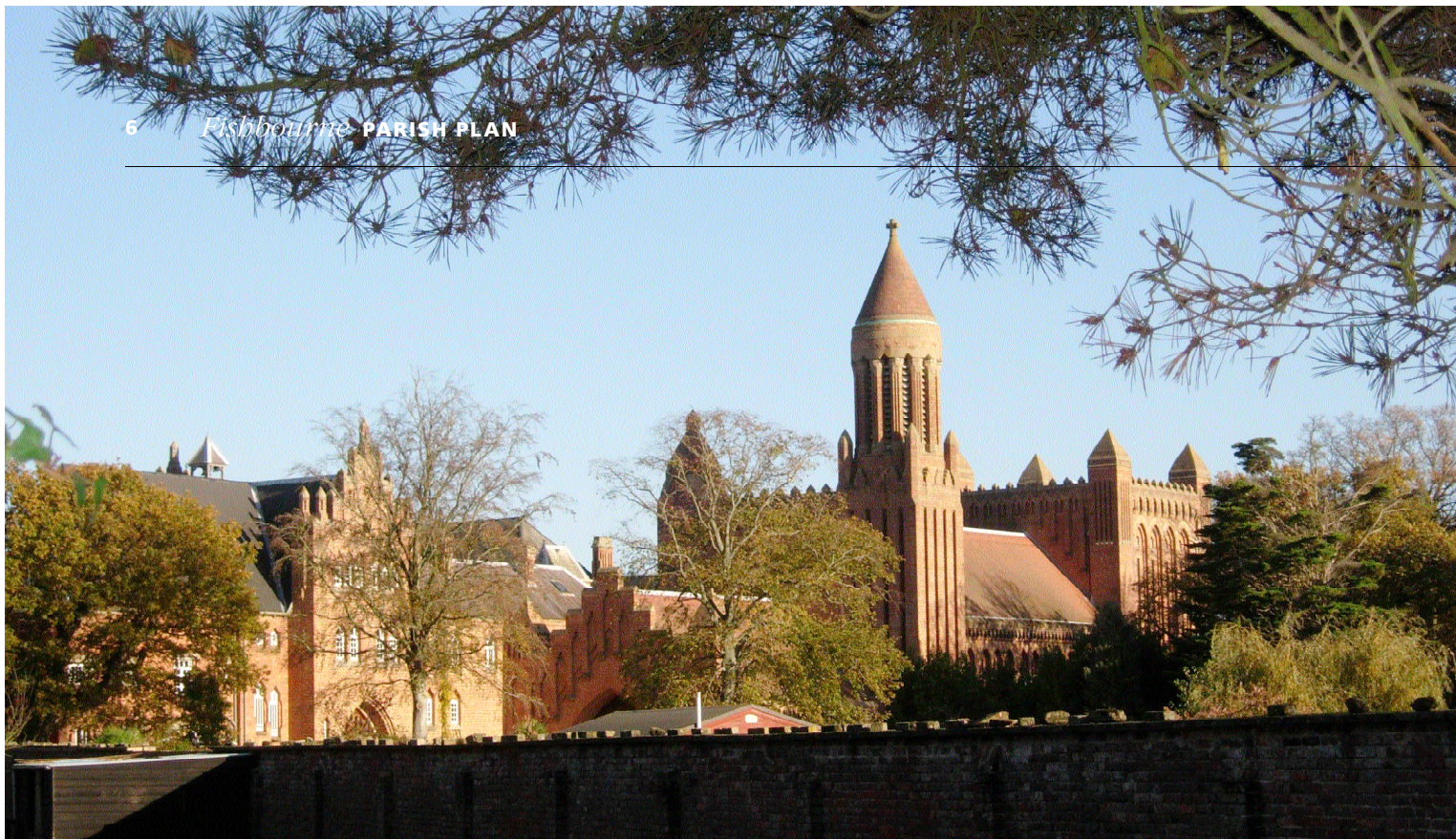
The Abbey church of St Mary, at Quarr. Work commenced in April 1911 and was finished in 1912. 300 tradesmen from the Isle of Wight were employed in its construction
