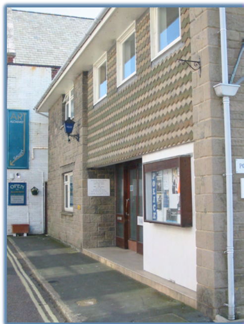
Yarmouth Police Station © BCE
