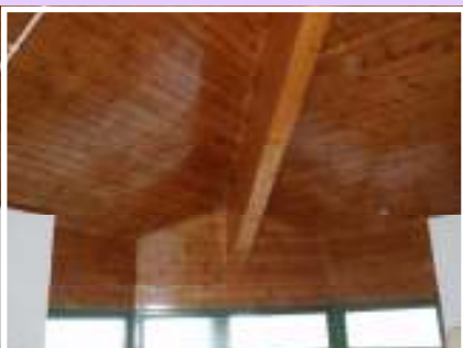
Refurbished health suite ceiling
