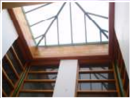
Atrium above changing room lobby
