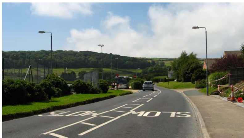
Works undertaken 2006/07 – Newport Road Ventnor (Safe Routes to School including carriageway repairs and new bus stop)
