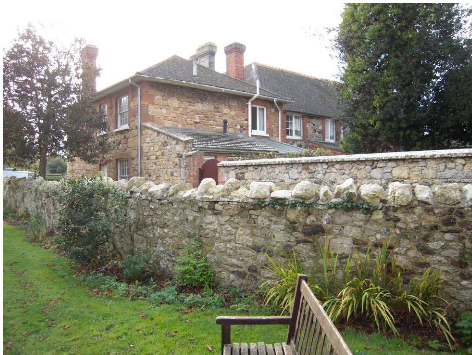
Figure 11: The rear elevations of White Cottage and the Red Lion
