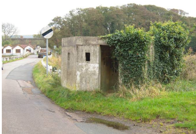
Figure 23: A hexagonal type 22 pillbox, which commanded the broad crossing of the River Yar and railway line.
