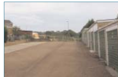
Existing garage court
